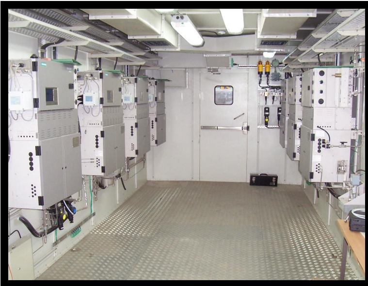
Gas Chromatographs inside Analyzer Shelter
